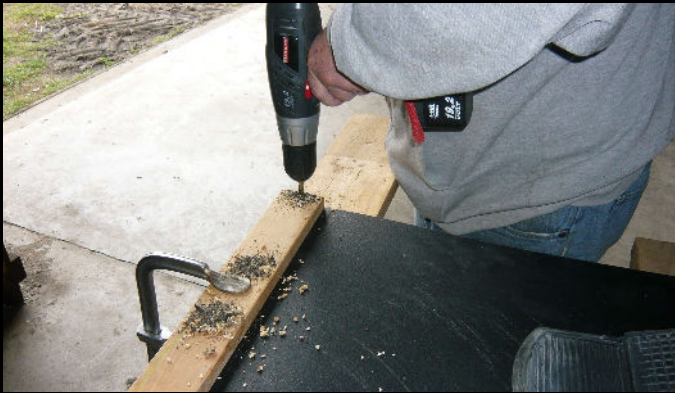
FIG. 1-3. Drilling the Holes
